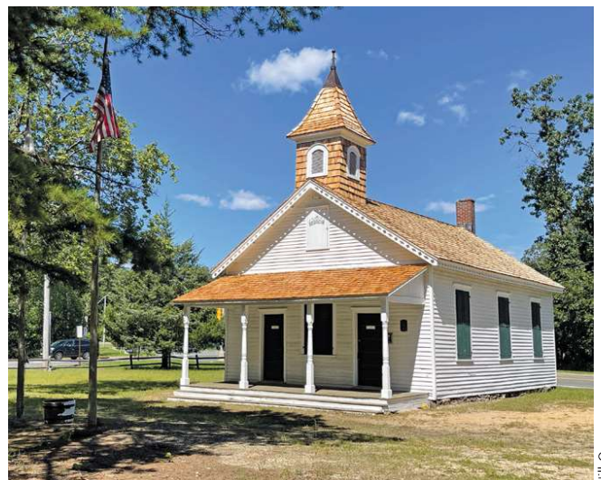
Georgia Road School House in Freehold.
