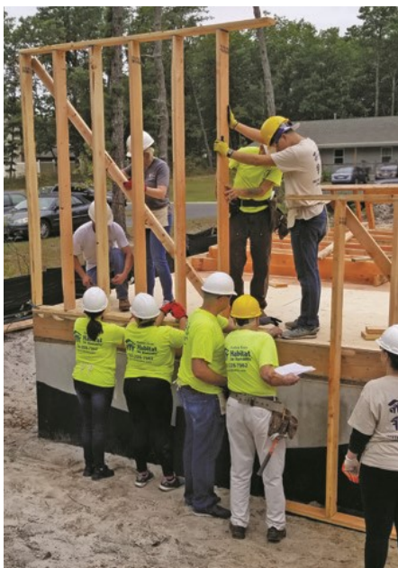
courtesy of Northern Ocean Habitat for Humanity
