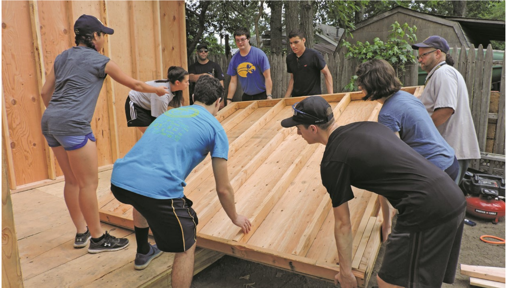
courtesy of Northern Ocean Habitat for Humanity
